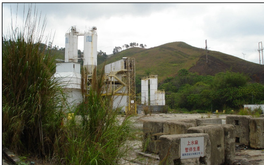
Photograph 2-4 View to the North – Concrete Batching Plant
